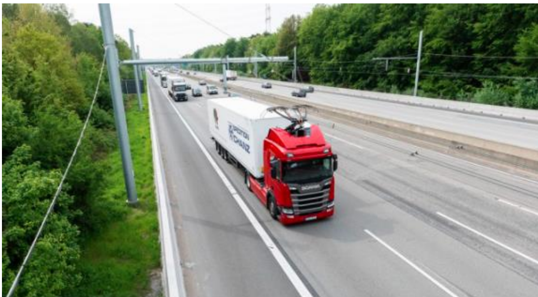
Figure 11 – Electrified road system trial 52
